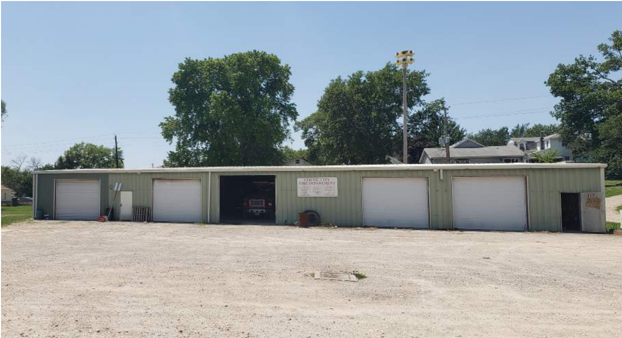
Existing building - East face
