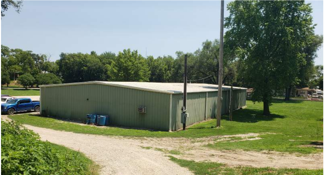
Existing building - North and West face
